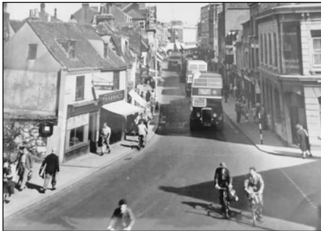
Biggin Street Before Widening
