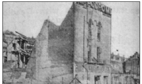
Demolition of the Hippodrome, 19th January 1951
