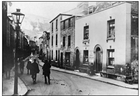
Limekiln Street Dover
