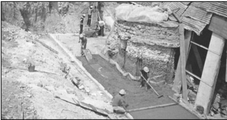
Roman Fort Work in Progress
